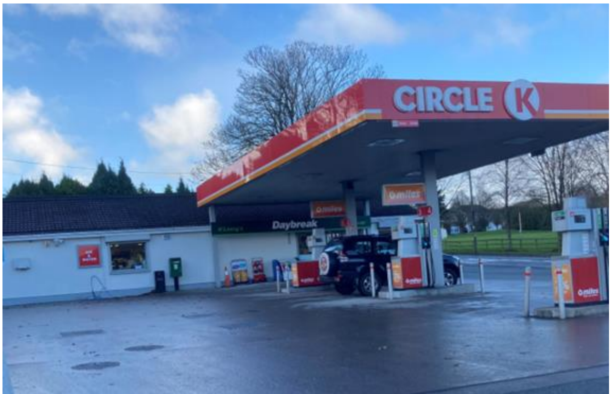
Figure 2.3 Circle K/Daybreak - Tower
